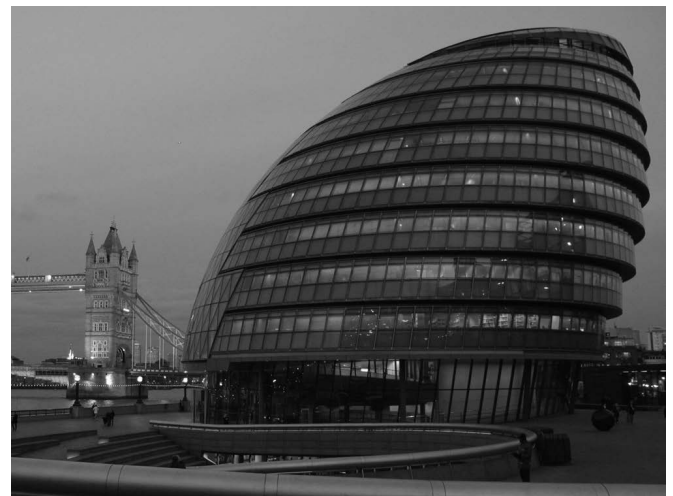
Fig. 3, the optimization of environmental parameters was the guiding principle to design the London City Hall, by Foster & Partners.
