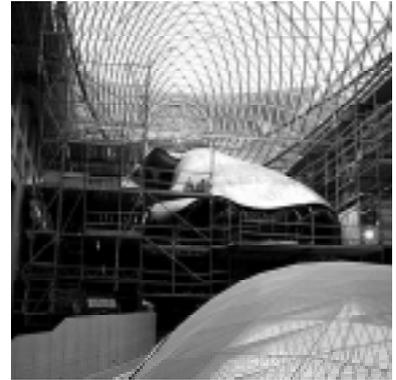
Fig 3. Glass envelope in Gehry's building in Berlin produced by triangulation.
