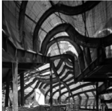
Fig 2. Structural frames in Gehry's building in Seattle produced by contouring.
