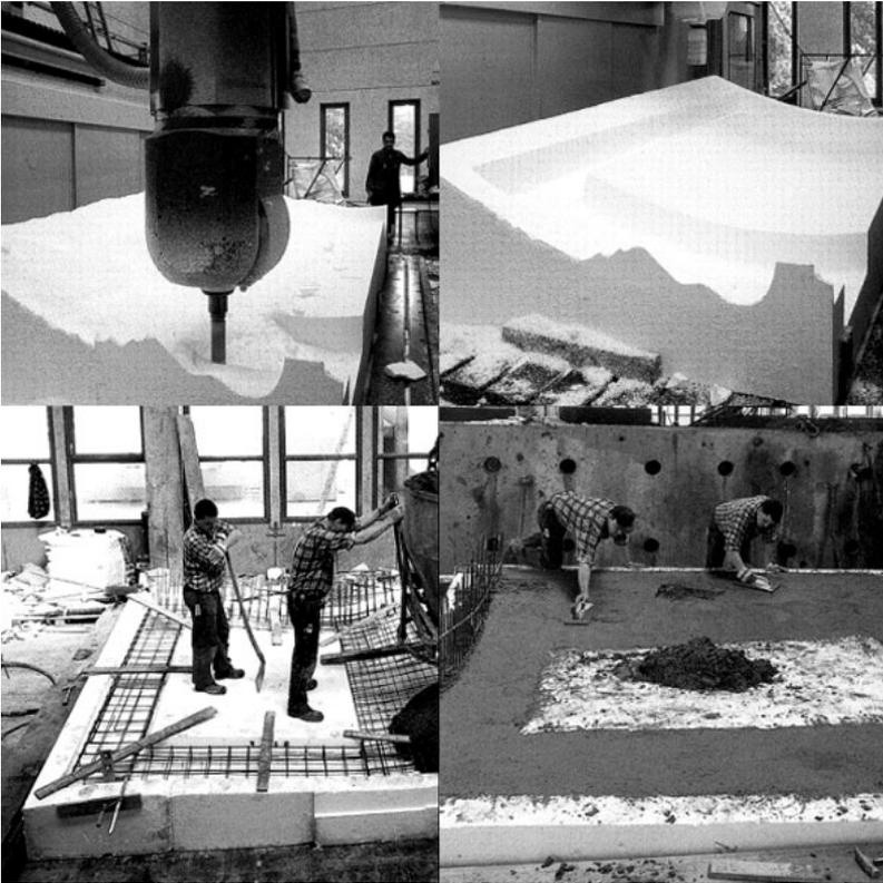
Fig 5. Milling of molds for concrete casting in Gehry's building in Dusseldorf.
