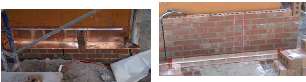
Figure 6 Augmentation of masonry wall ties in CMU backing wall
