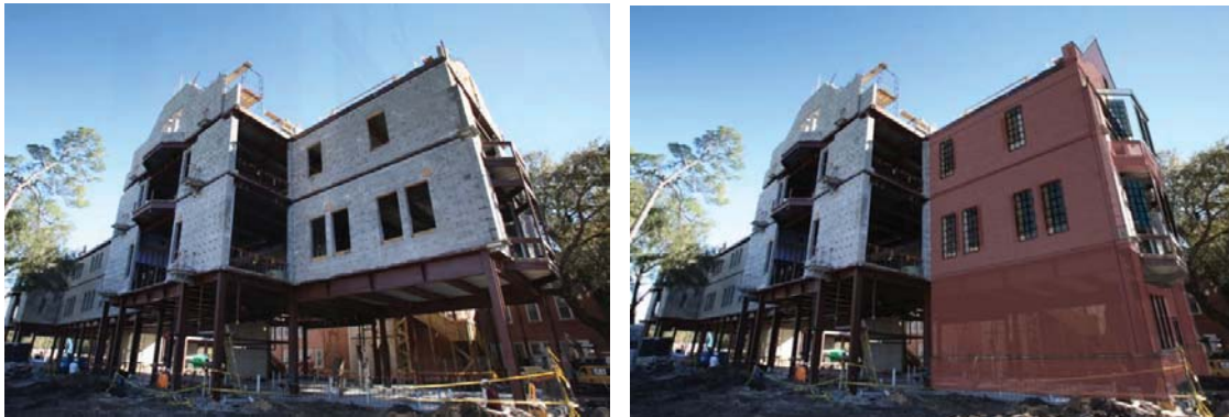
Figure 3 Completed BIM model augmentation over on-site construction progress documentation
