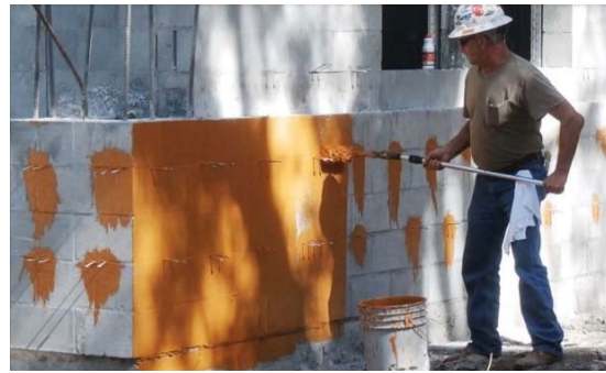
Figure 2 Example of project documentation, waterproofing installation on the exterior CMU
