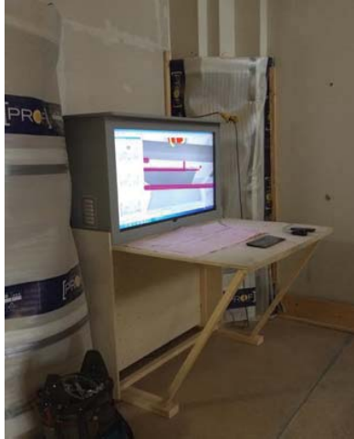
Figure 1 BIM kiosk located at the construction site
