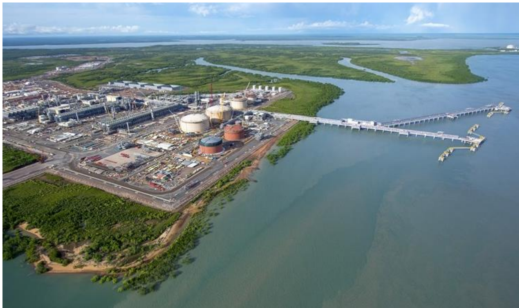
Figure 1 Overview of Ichthys LNG Project construction site (INPEX Australia 2016)
