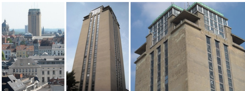
Fig. 1: (left) the tower in its urban fabric pictured from the top of the Belfry; (right) two views of the Book Tower from the street. (Source: personal archive of the authors).
