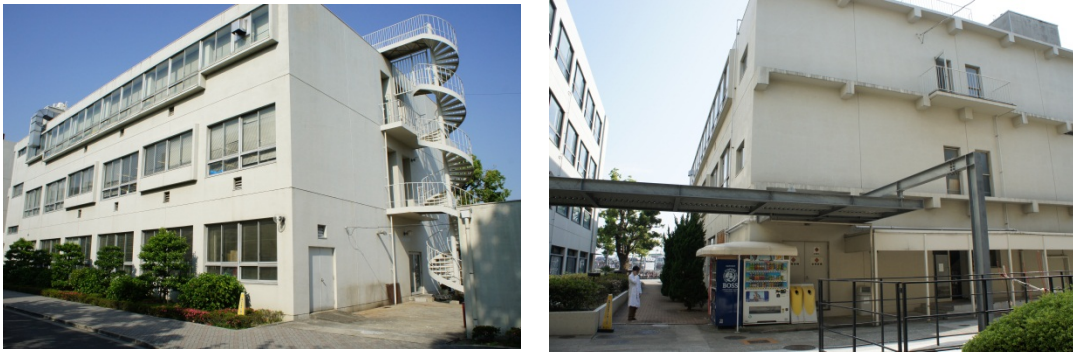
Fig. 11: On-site photos; there are some obstacles for practical scanning
