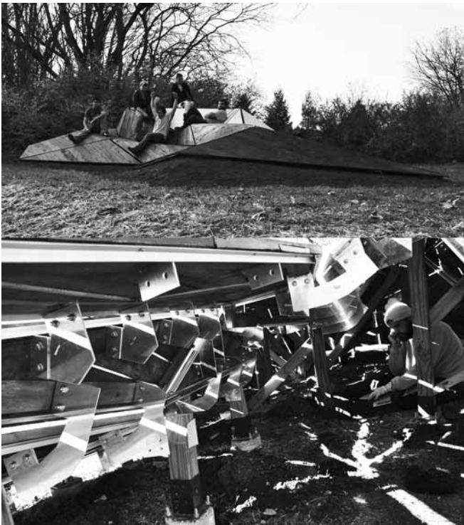
Figure 4. ReBarn: assembly and occupation (Zahner Metals tooled aluminum and barn siding)
