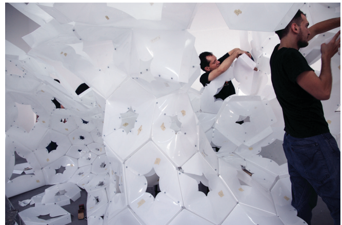
Figure 11: Assembly of the pavilion.
