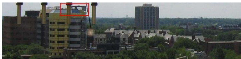
Fig. 4: UM Central/Medical campus School of Public Health construction site identified as highest point
