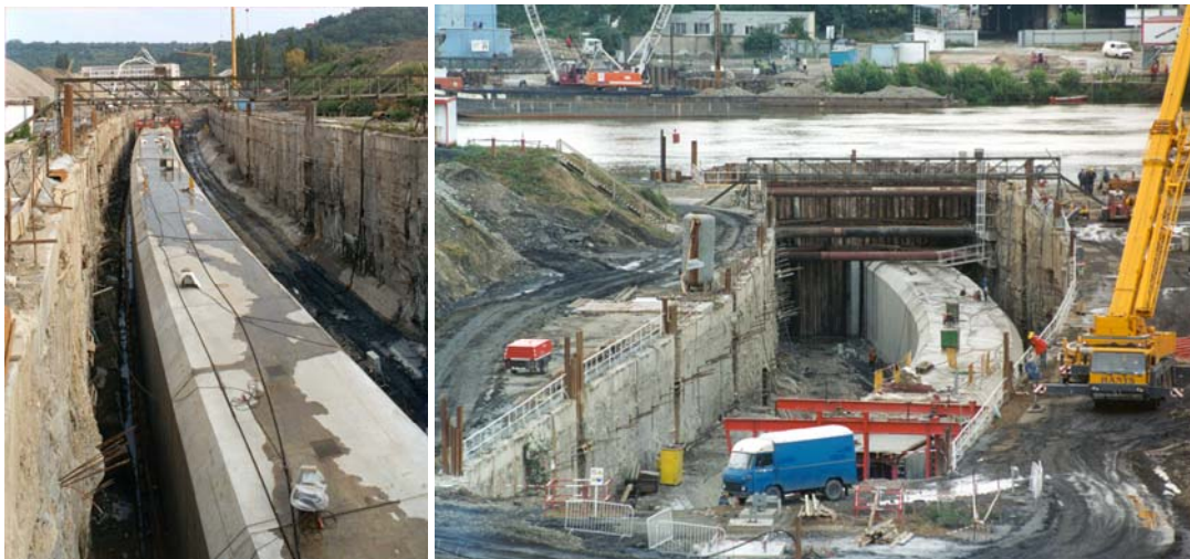
Figure 1: A Subway Tube in Dry Dock (left) and after Launching
