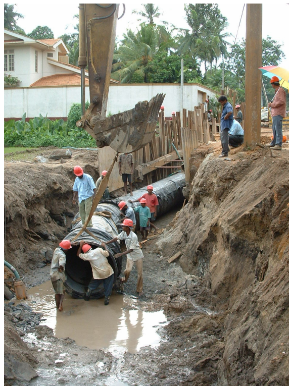
Figure 5. Construction work on site.
