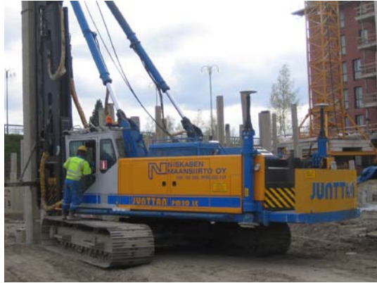
Figure 4. Junttan PM-20 piling rig.
