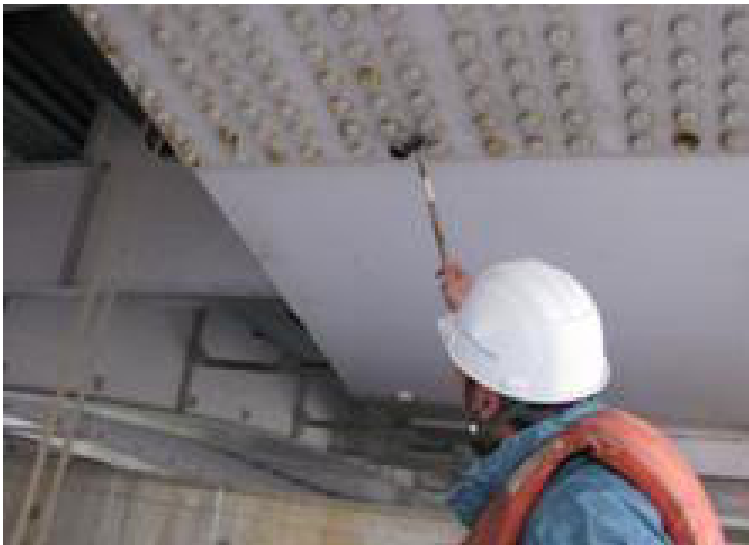
Figure 5. Inspection works for bridge
