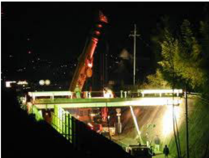
Figure 4. Crane works for one span bridge
