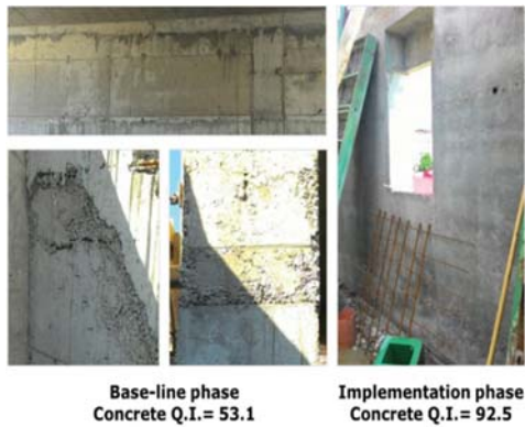
Fig. 8 – Comparison of the quality of concrete works between the two phases of the study
