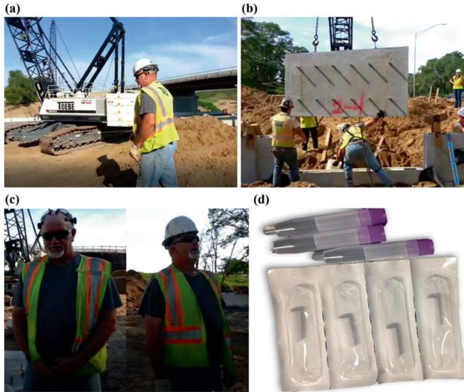
Fig. 21.3 EEG data collection in field: a Low stress experimental tasks (e.g., working on the ground level and working right after break); b High stress experimental tasks (e.g., working at top of a ladder, working in a confined space, and working in dangerous environment); c Wearable EEG headset fit into worker's safety hardhat; d Salivary cortisol samples kit
